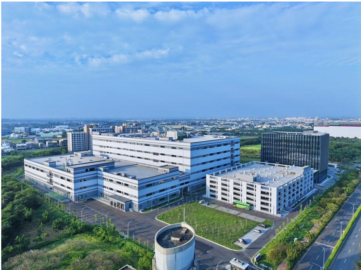
Note: Kaohsiung AI Park Site Overview
